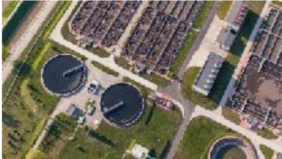
Sewage and water treatment
